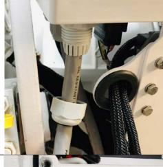
12. Check that cable gland is completely secure and that there is no void between the cable and gland.
