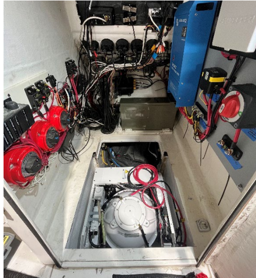
Figure 4: Seakeeper Installation and Final Wiring
