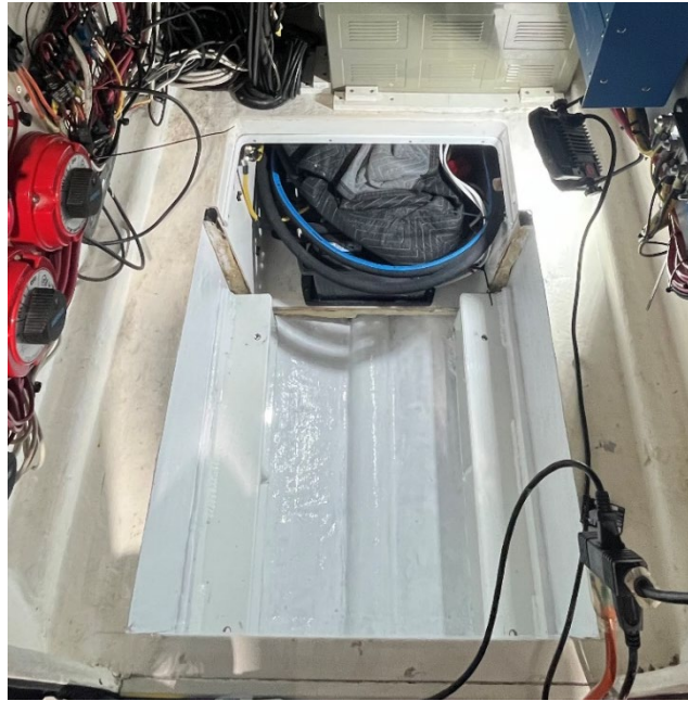
Figure 2: Final Installation of Seakeeper Mounts
