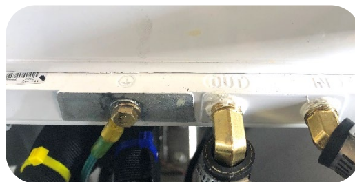
Motor drive ground connection
