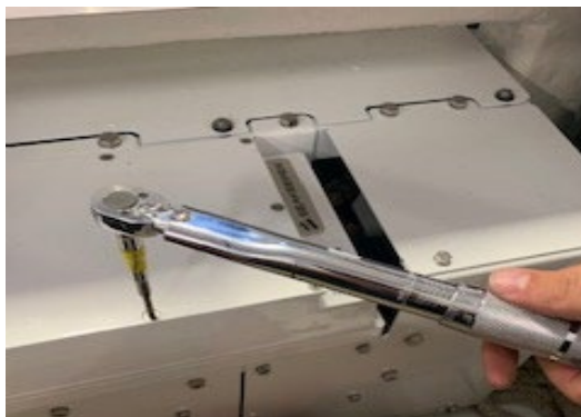
Figure 42: Torquing AC MDB cover screws
