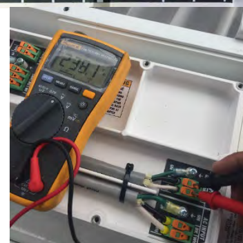
Testing SW Pump voltage
