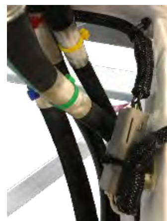
Photo showing location of Guide Band connector inside foundation near guide band bracket and below manifold.
