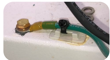
Figure 15: Example of heat exchanger ground cable to foundation
