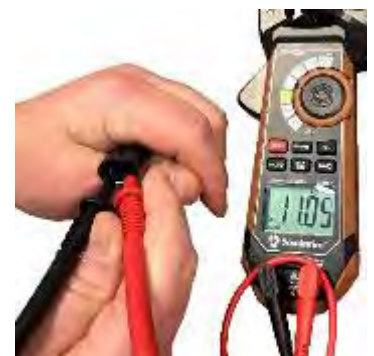
Meter in this photo is displaying 11.05 KΩ.
